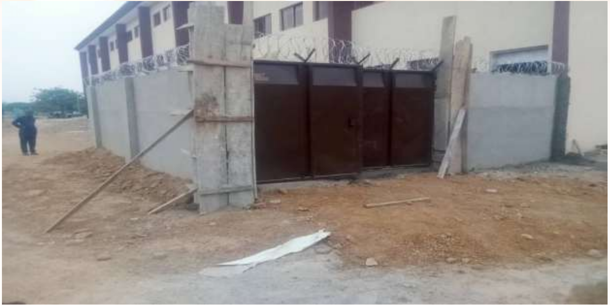
Construction of Grave Yard
