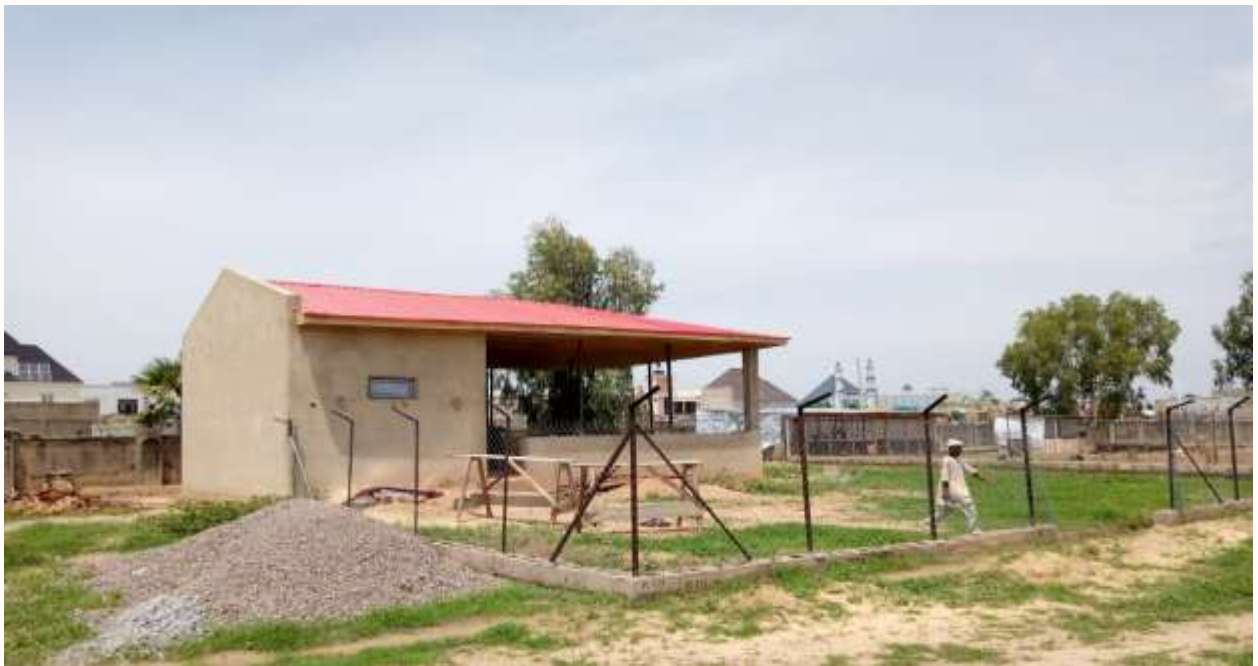
Construction of Animal Shed at the Entrepreneurship Poultry House
