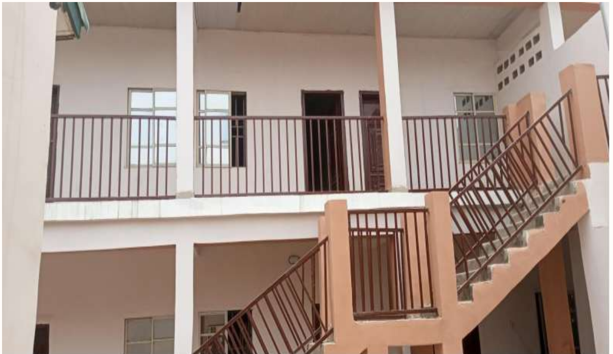
Figure (43): General Paint Renovation works for the Additional 16no of students' hostel Rooms allocated to the University at MMSH
