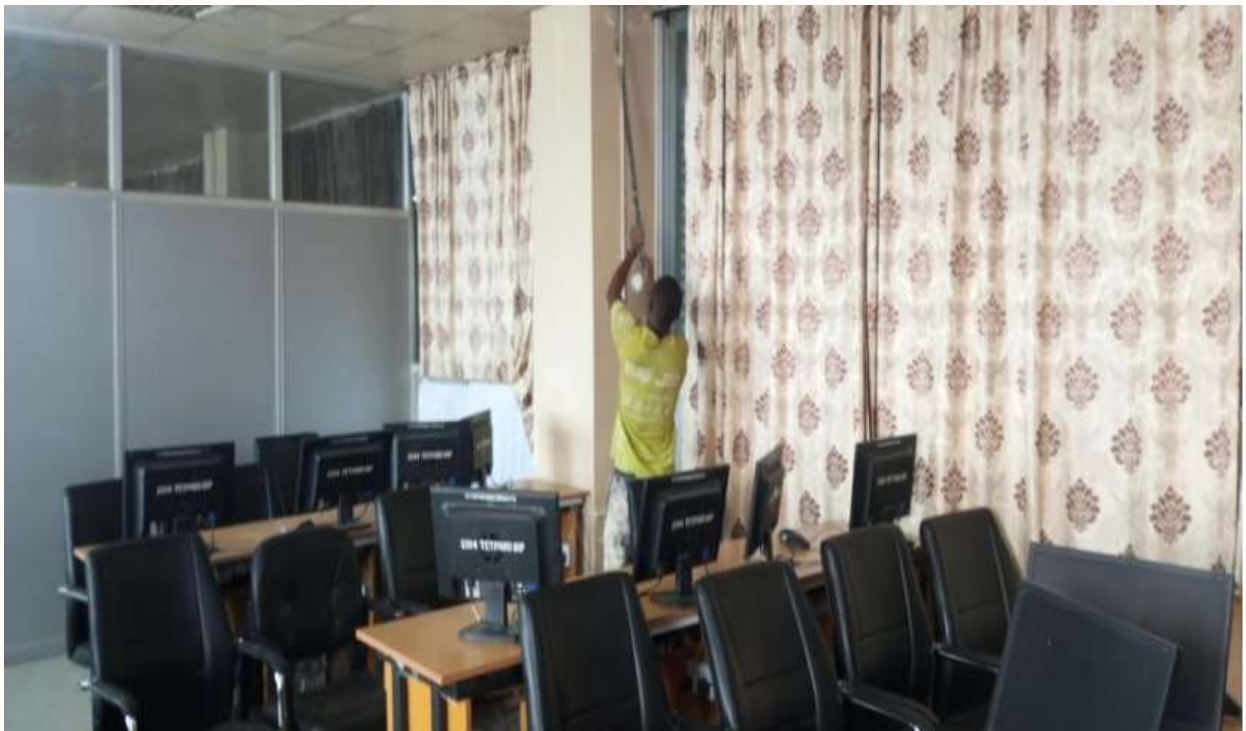
Figure (32): Renovation works at 9 th and 10 th floors, City Campus
