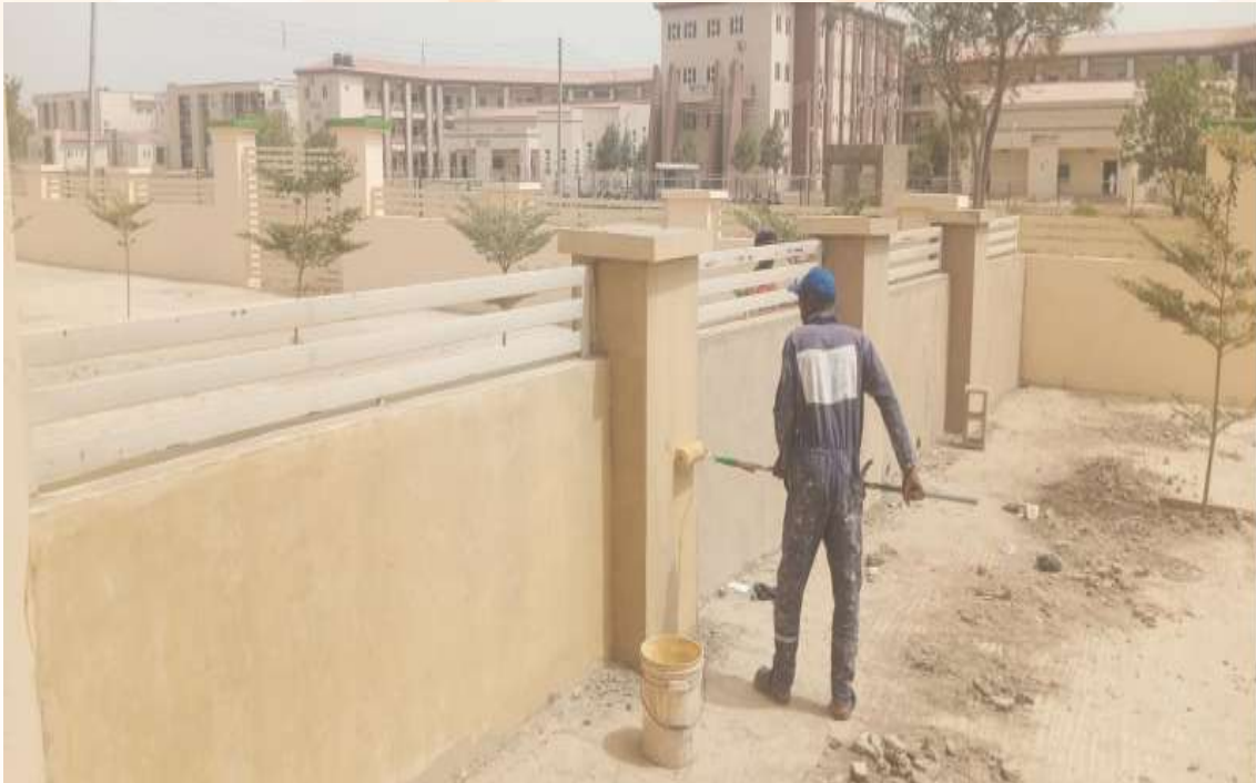
Figure (17). Construction of fence for the demarcation of male and female sections at the newly constructed mosque at Academic area, Main Campus
