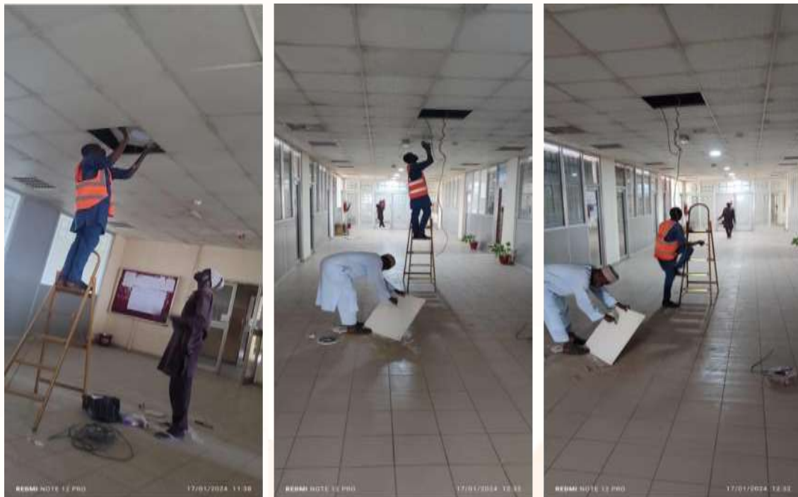
Figure (8). Replacement of dead lightning bulbs at the 7 th Floor Library, City Campus
