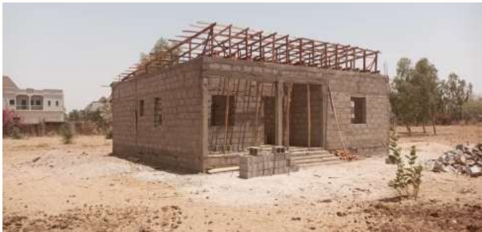
Ongoing construction of Animal House by TETFund
