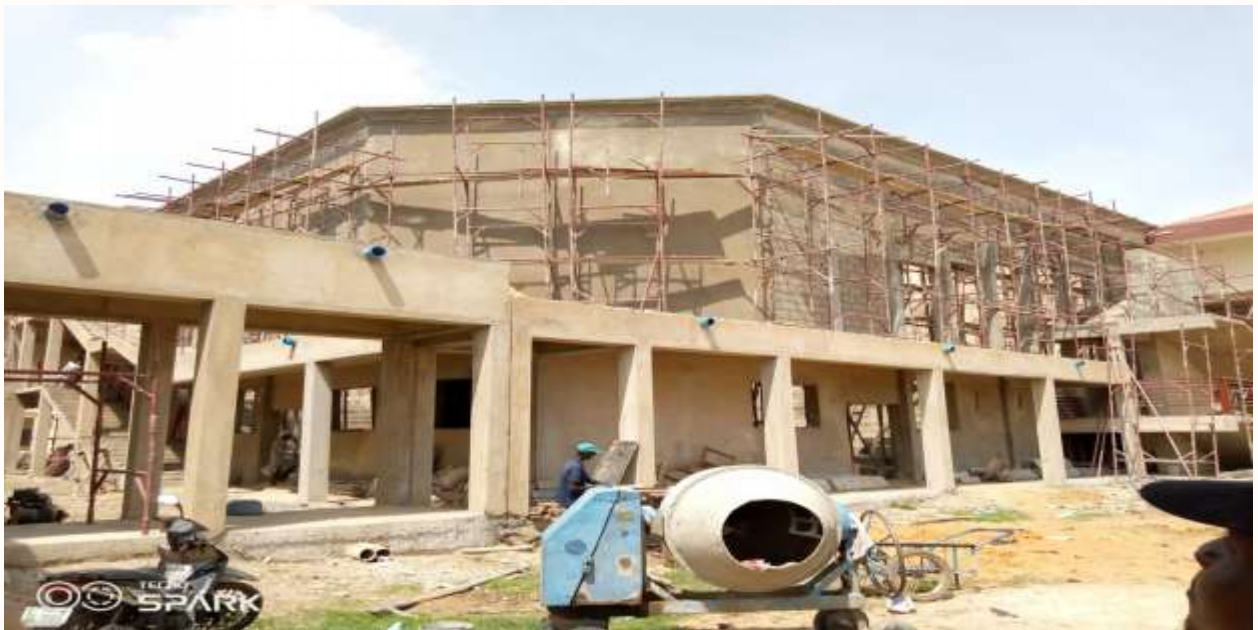
Completion of 3no. 500-seat Lecture Theatres at the Faculty of Science
