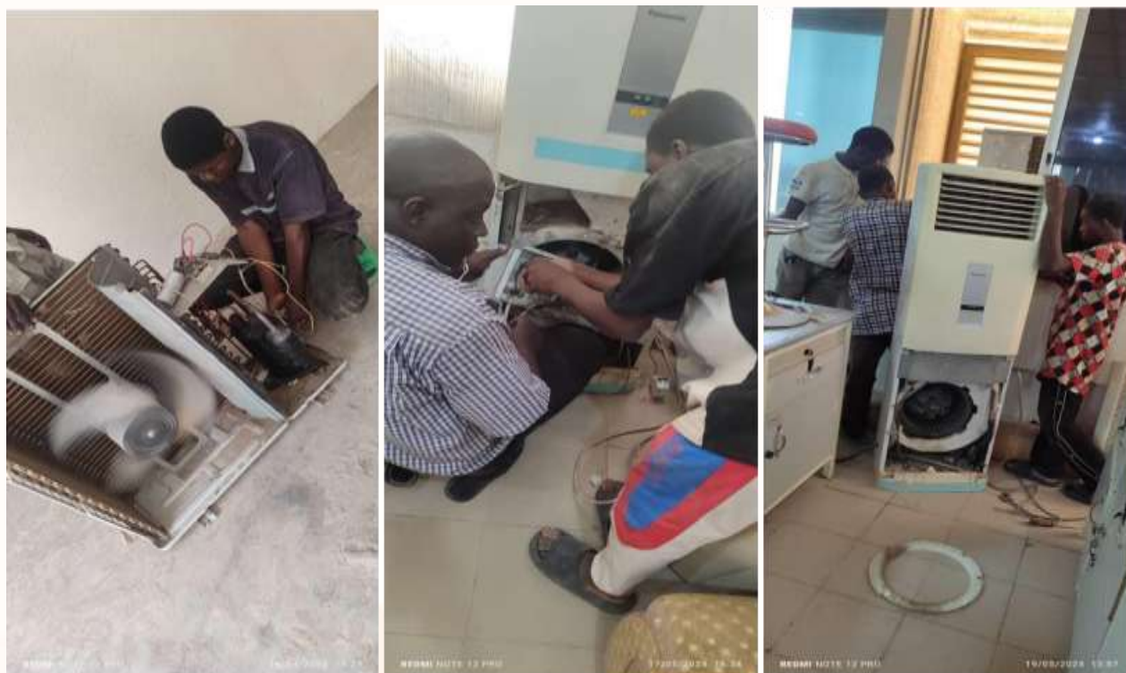
Figure (2). Repairing of Air conditioners at Multipurpose Laboratory, 6 th floor, City Campus
