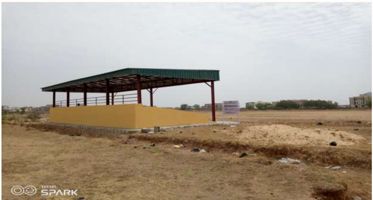
Completed Sports Pavilion
