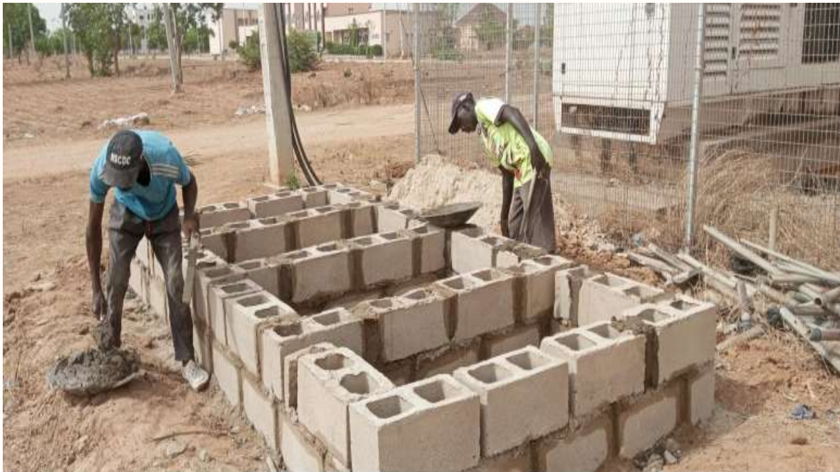
Figure (40): Construction of Generator base at Main Campus
