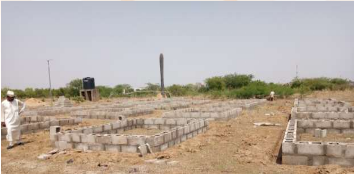
Construction of nursery bases at the Botanic Garden
