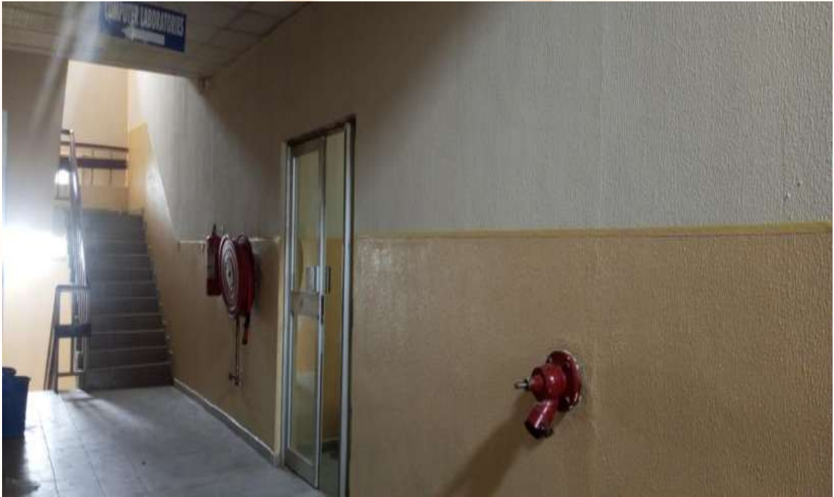
Completed Paint Renovation works at 6 th , 9 th and 10 th floors, City Campus
