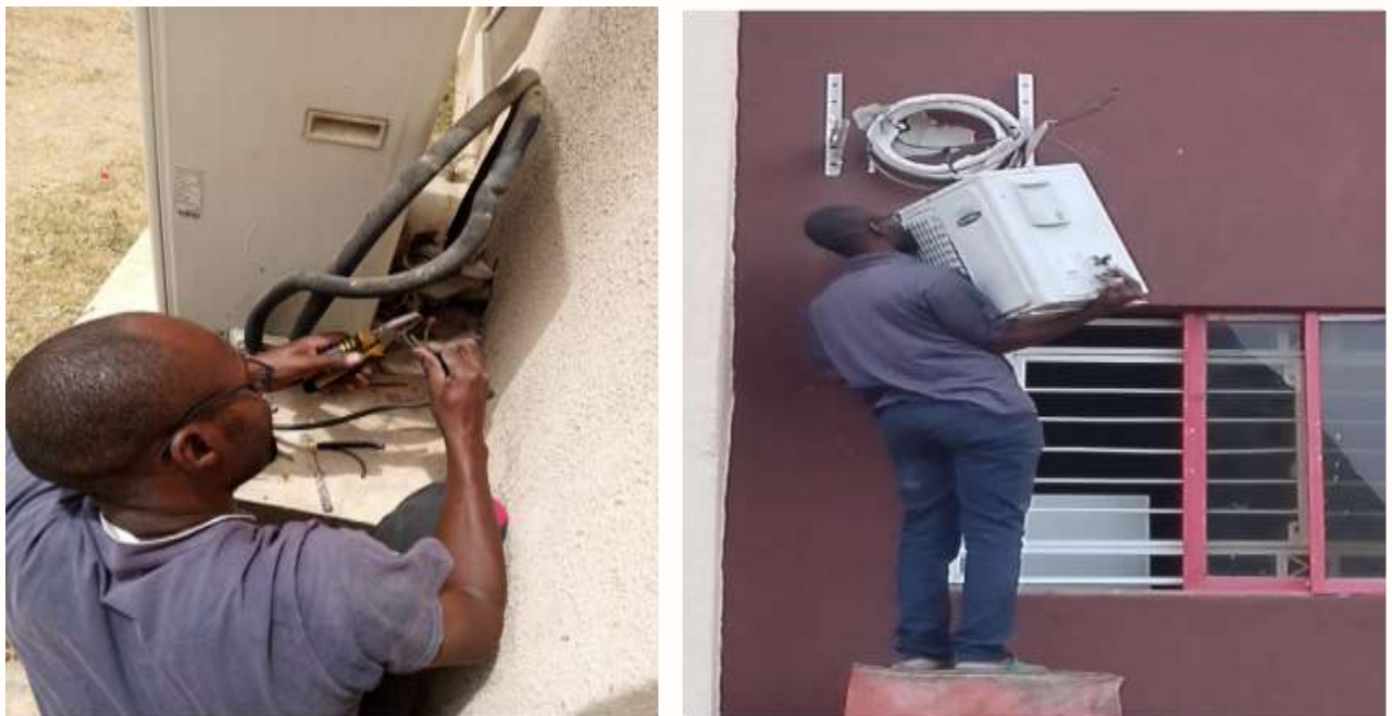
Figure (10). Installation of 23no.s of air conditioners at 4no.s of Laboratories, Staff Offices and Animal house, Faculty of Basic Medical Science, Main Campus
