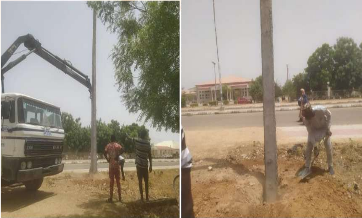
Figure (15). Replacement of pole at the Main Campus
