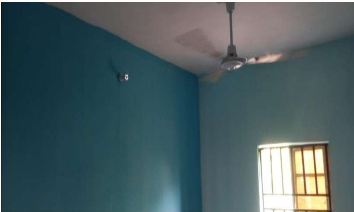
Figure (42): General Paint Renovation works for the Additional 16no of students' hostel Rooms allocated to the University at MMSH
