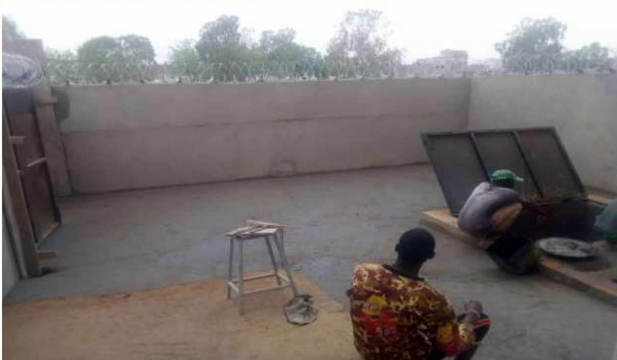
Construction of Grave Yard
