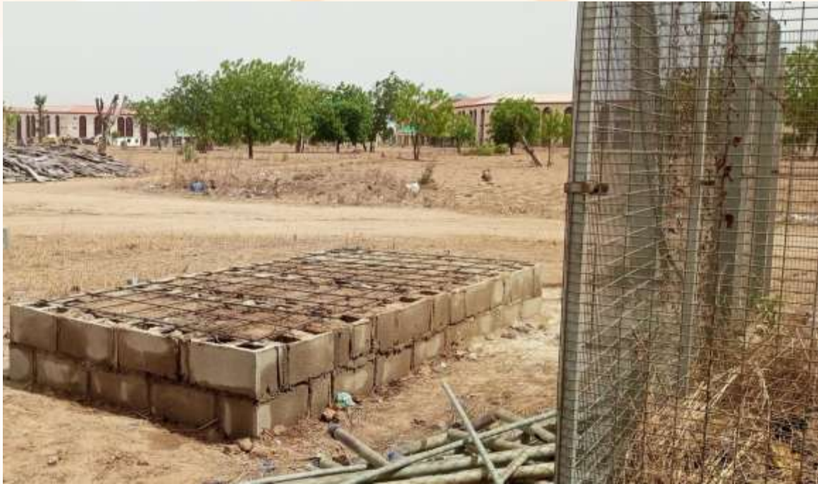
Figure (41): Construction of Generator base at Main Campus
