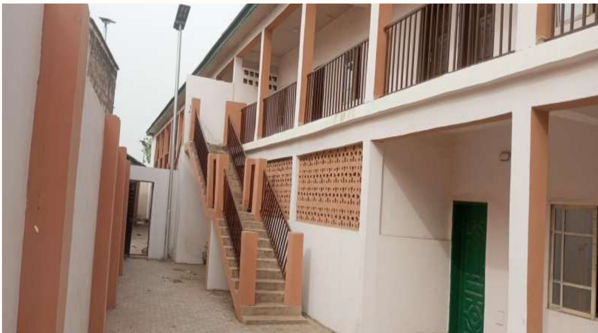
Figure (44): General Paint Renovation works for the Additional 16no of students' hostel Rooms allocated to the University at MMSH
