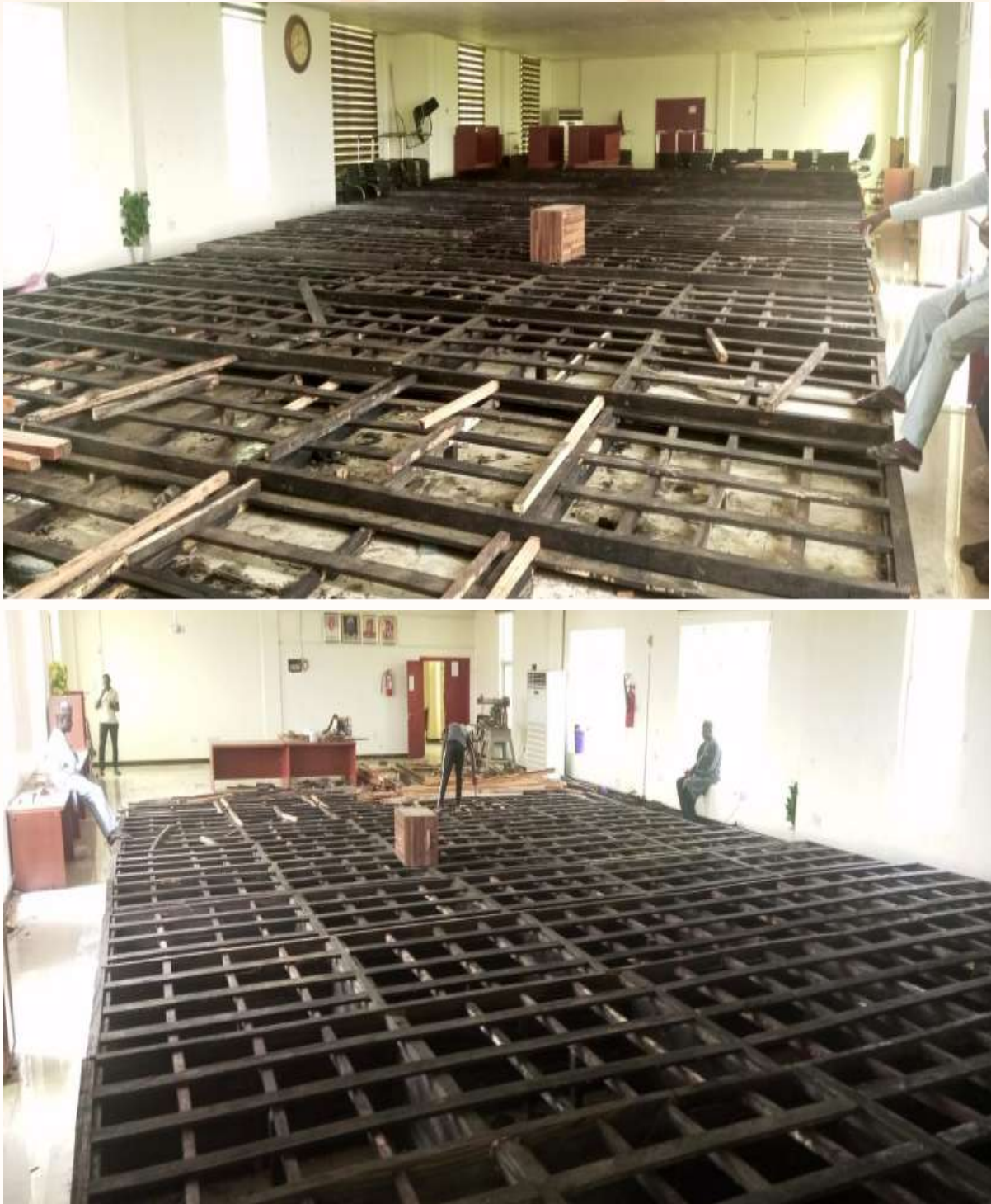
Figure (53): Design and Supervision for the Modification of Senate Chamber Seating Arrangement at Main Campus
