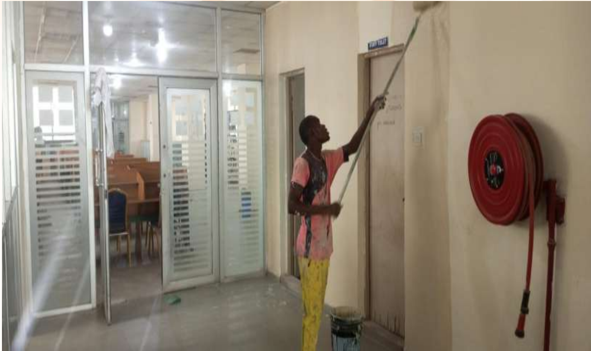
Figure (30): Paint renovation works at 6 th , 9 th and 10 th floors, City Campus
