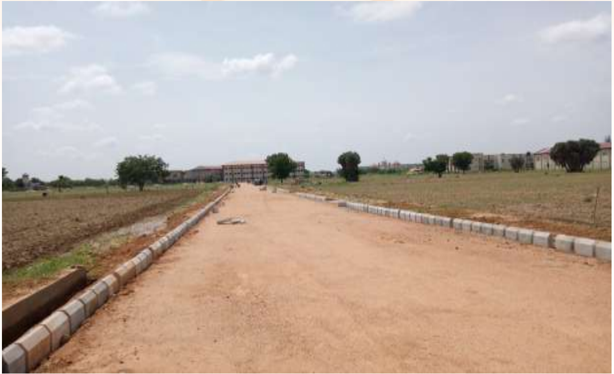
Construction of Internal Roads at the Main Campus
