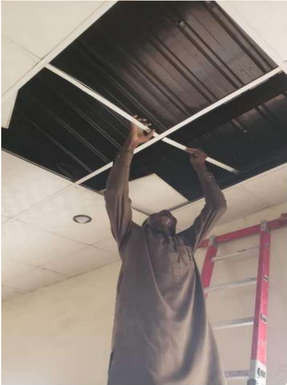
Figure (52): General replacement of broken door and window glasses, replacement of failed ceiling roof, collapsed suspended ceilings and welding of students' seat at various lecture rooms at City Campus
