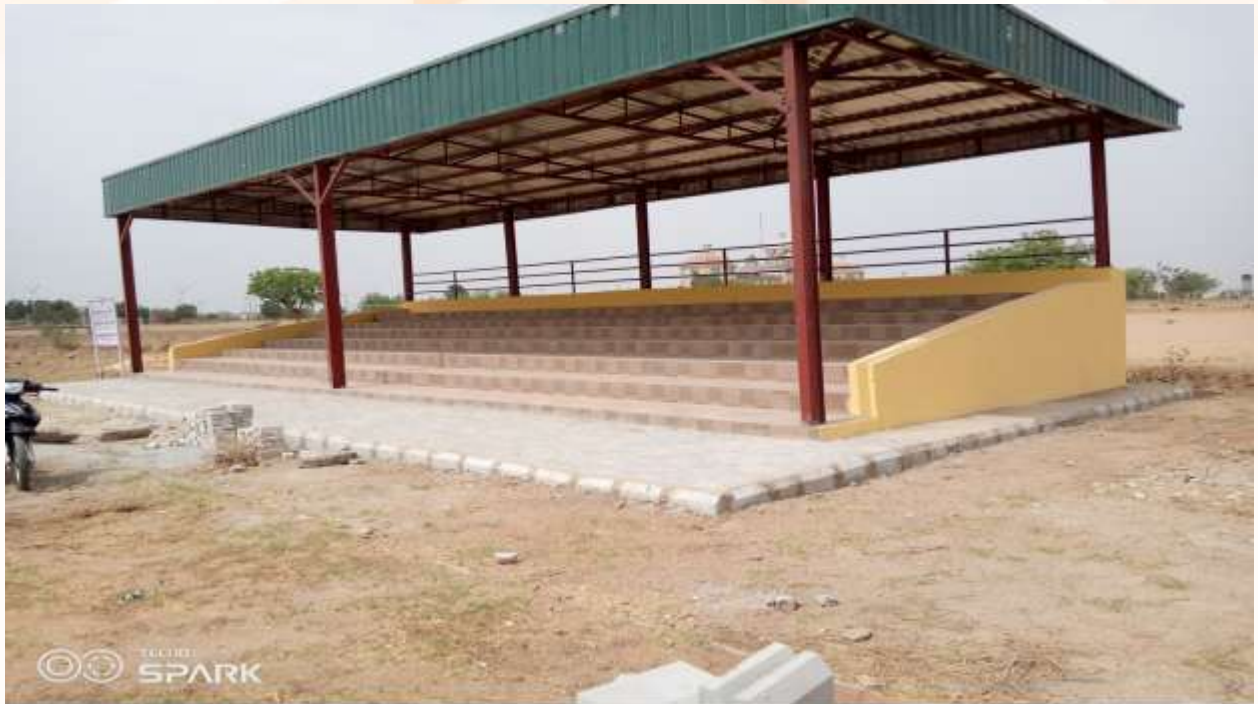
Completed Sports Pavilion
