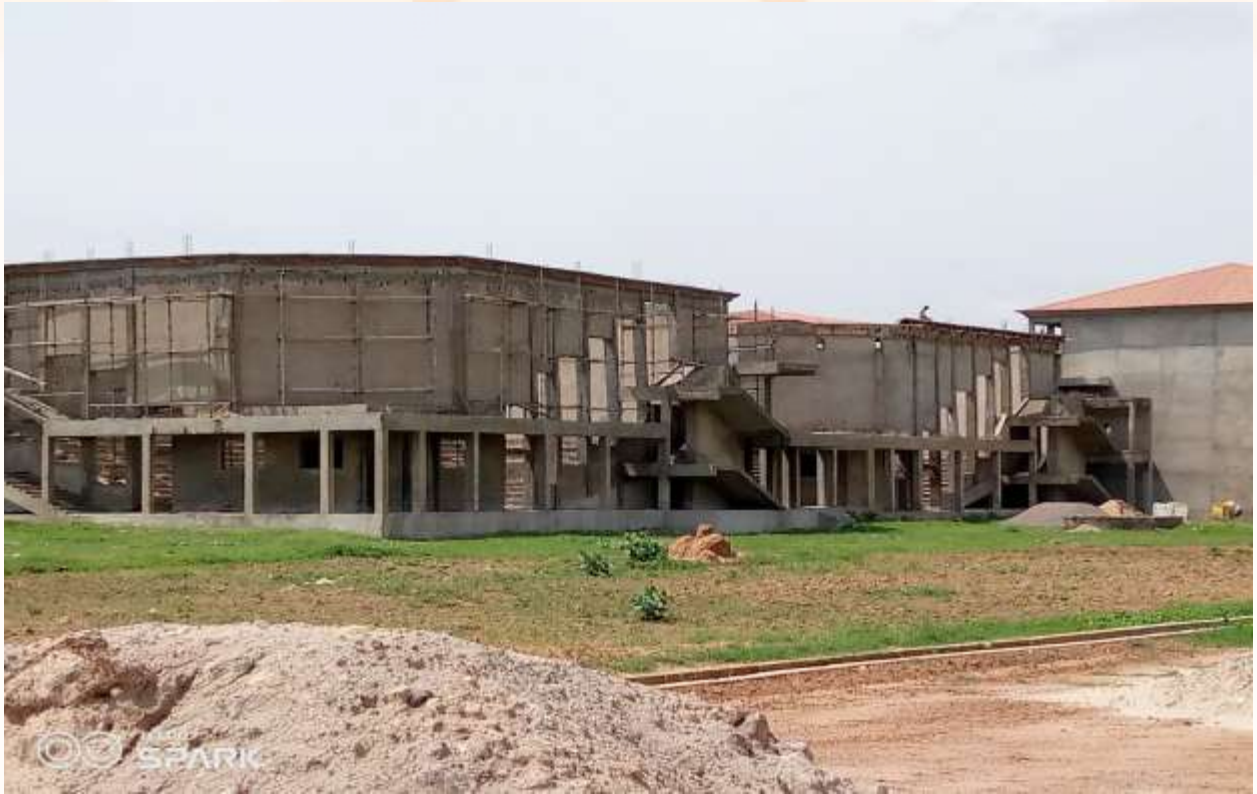
Completion of 3no. 500-seat Lecture Theatres at the Faculty of Science
