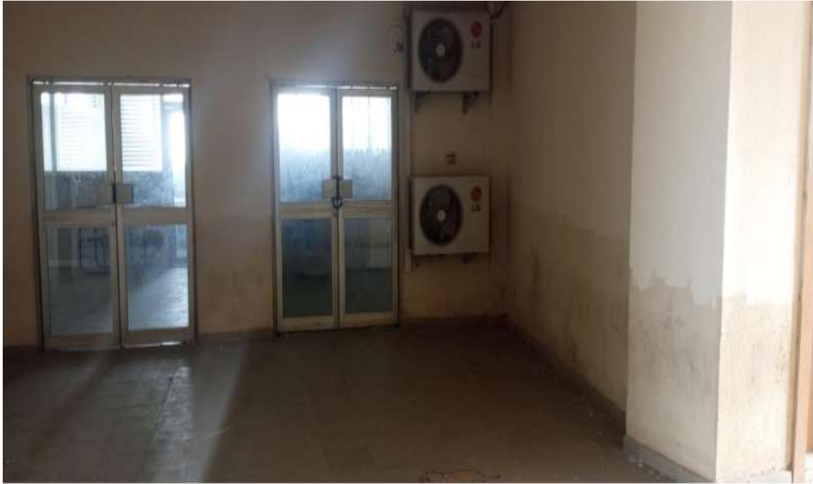
Figure (38). Paint Renovation works at 6 th , 9 th and 10 th floors, City Campus
