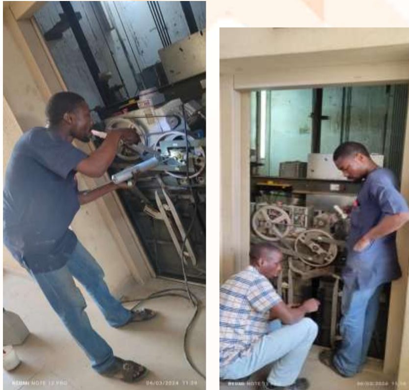
Figure (9). Repairs and Maintenance of Elevator at the City Campus
