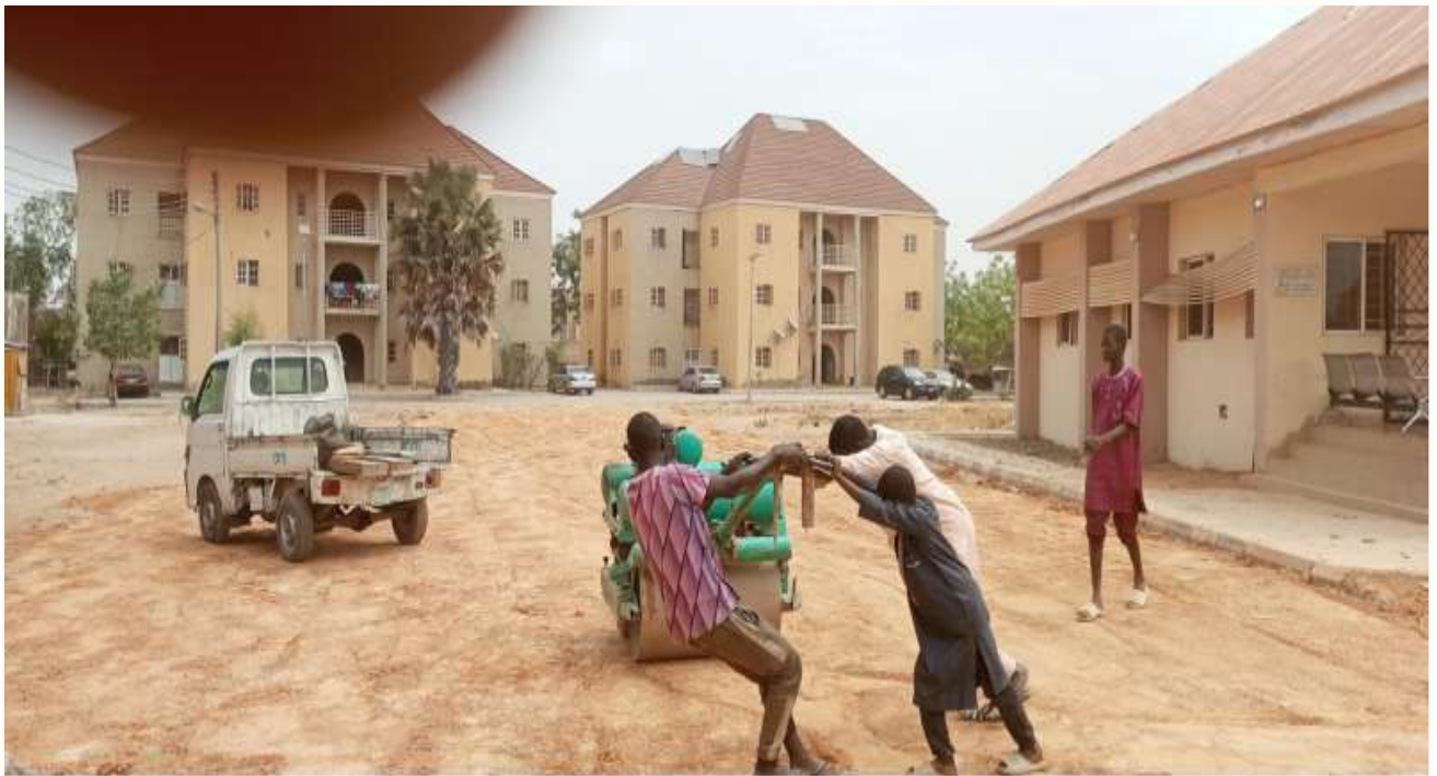
Supplying, grading and compaction of laterite soil at the Staff Quarter's access road
