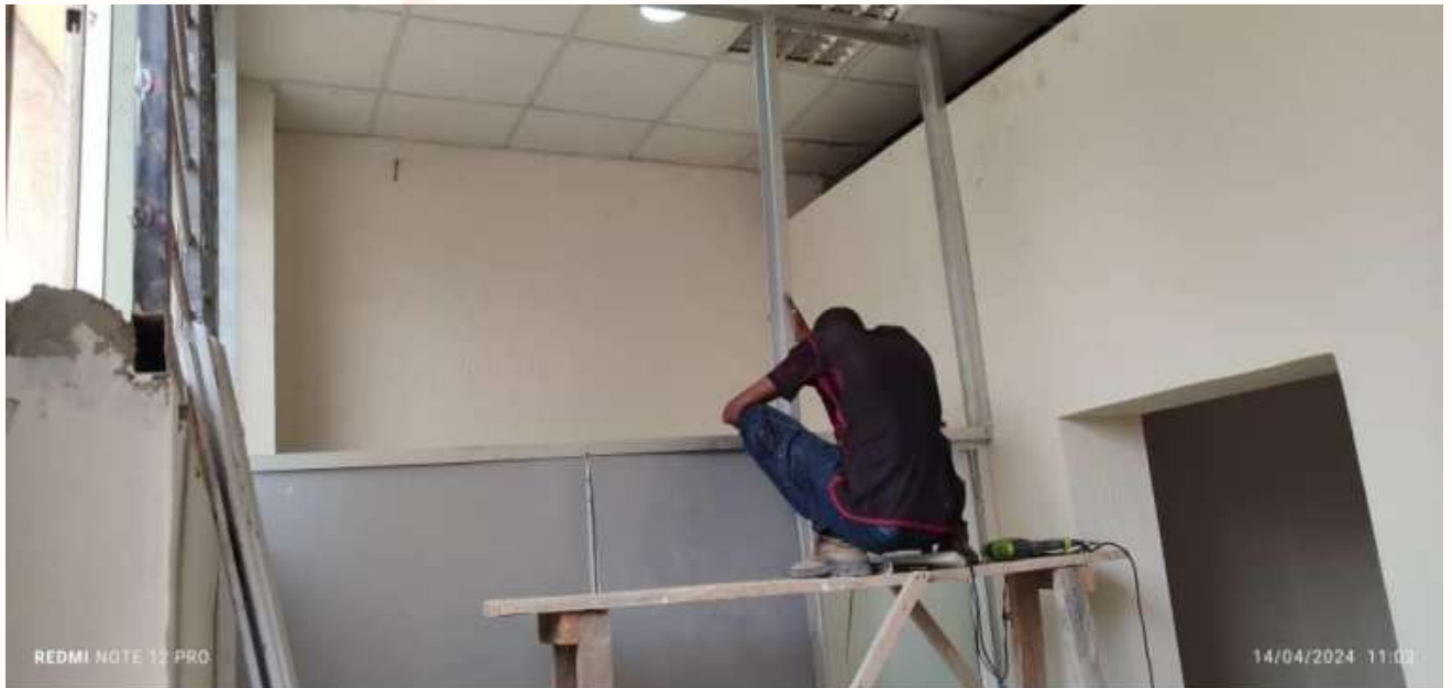
Figure (3). Renovation and conversion of Garage to the University Store at the City Campus
