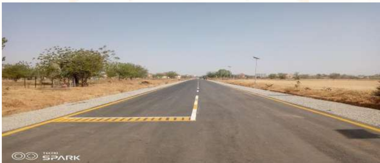
A picture of one of the completed roads at the Main Campus
