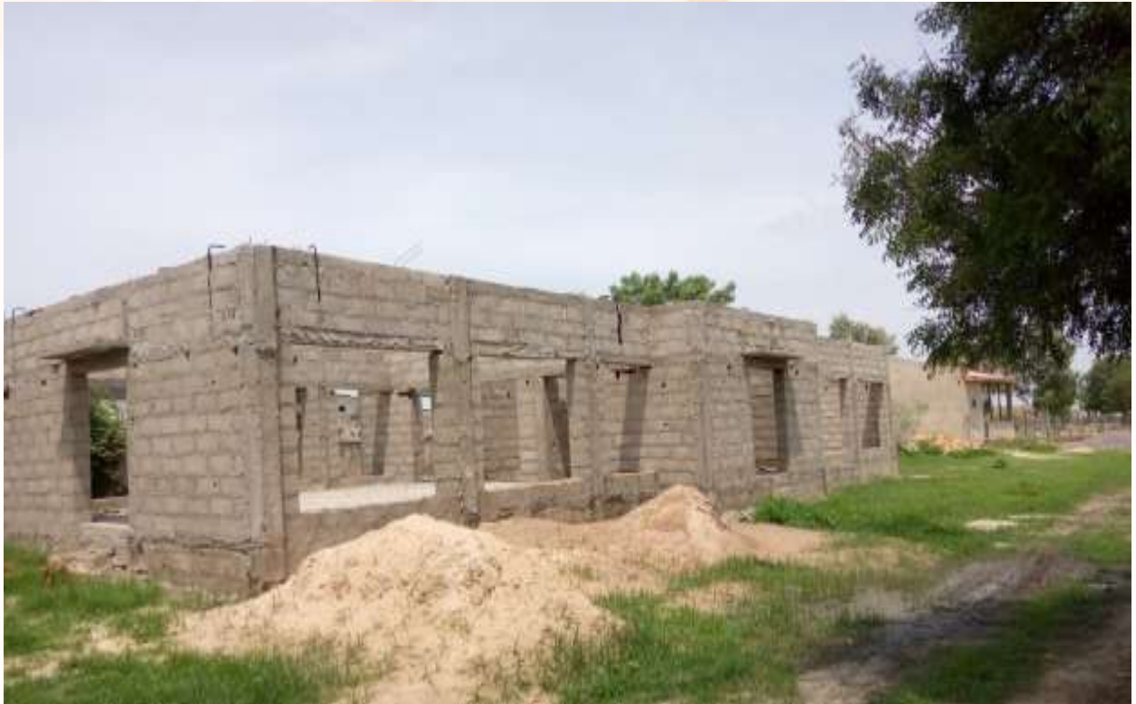
Construction of Brooding Hall at the Entrepreneurship Poultry House
