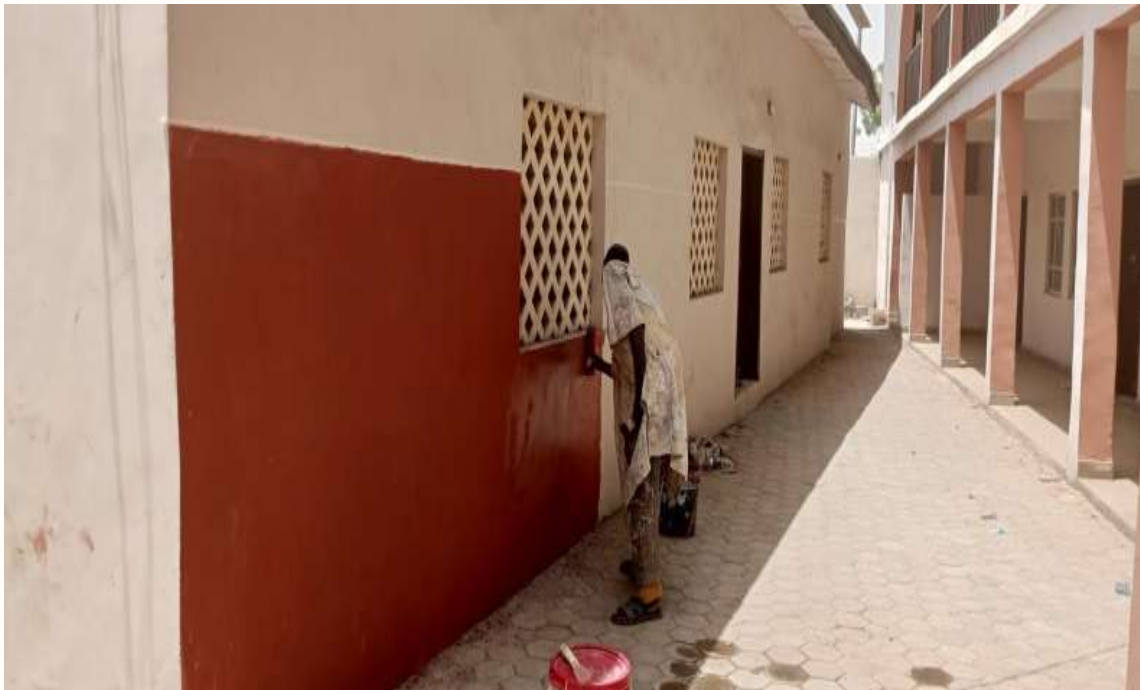
Figure (45): General Paint Renovation works for the Additional 16no of students' hostel Rooms allocated to the University at MMSH
