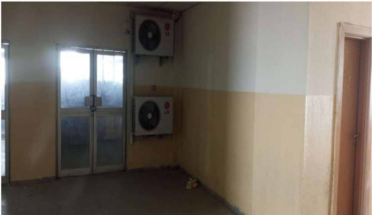
Figure (39). Paint Renovation works at 6 th , 9 th and 10 th floors, City Campus
