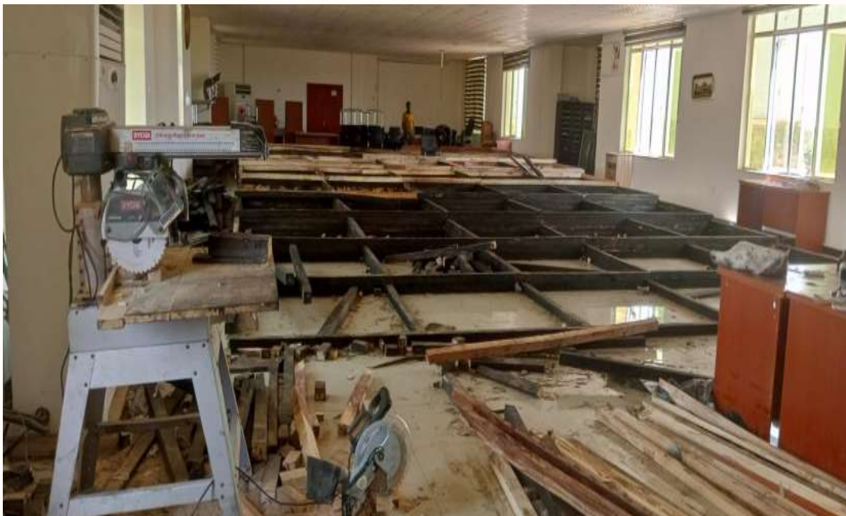
Figure (53). Design and Supervision for the Modification of Senate Chamber Seating Arrangement at Main Campus
