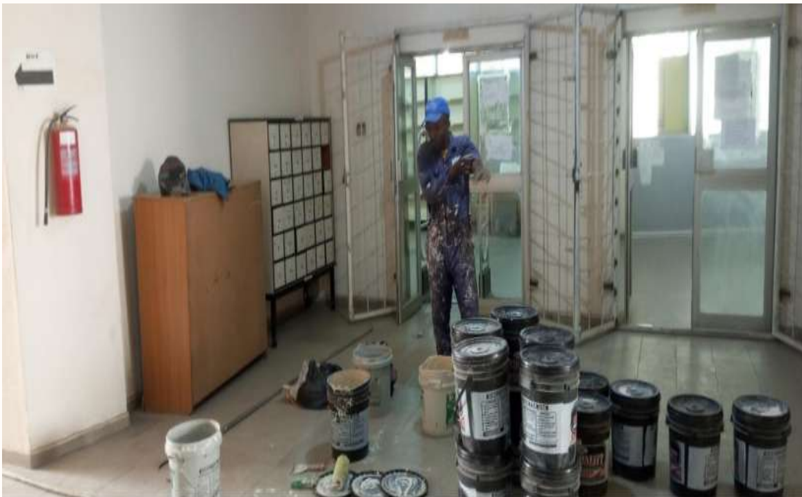
Figure (31): Renovation works at 9 th and 10 th floors, City Campus
